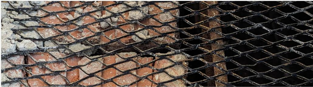
The full restoration of the wall will take at least another month to complete. This includes creating a uniform structure of restoration appropriate material across the length of the wall to reduce cracking. Then the painting of the new plaster will include the techniques of glazing, ragging, stippling, and dry brushing to match the original paint.
