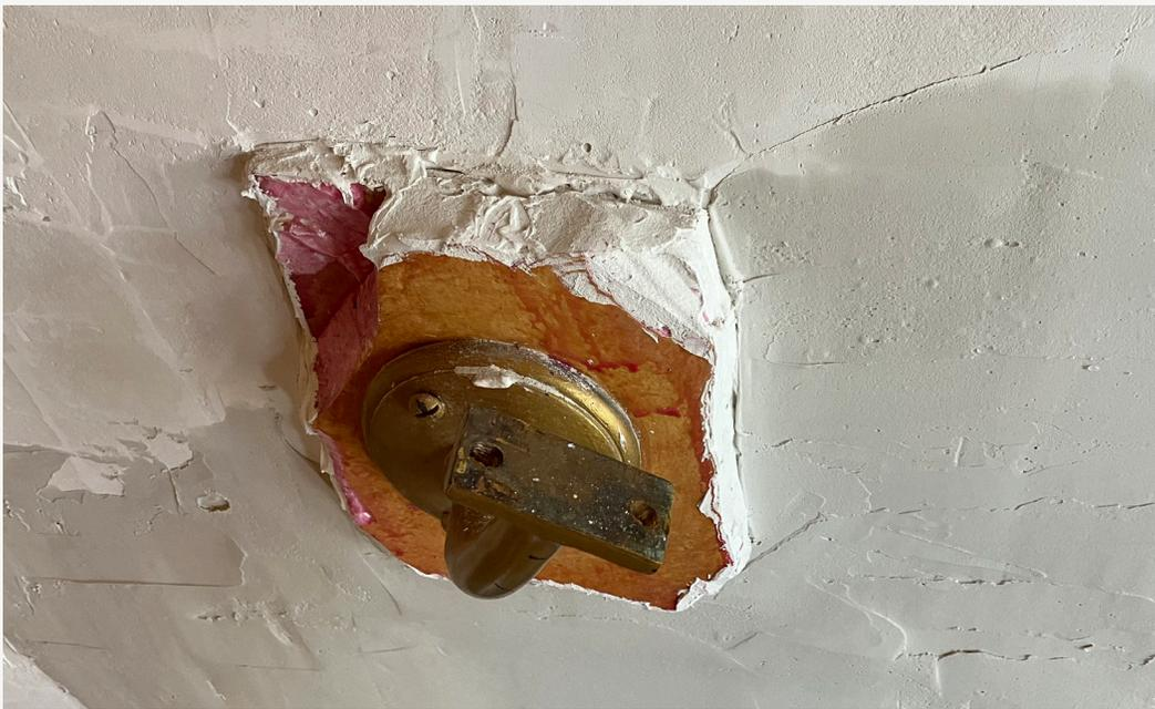
The raised area near the handrail displays the original depth of the wall. Layer upon layer of plaster was applied to match the original thickness.
