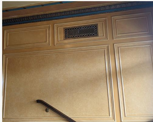
The 2nd floor men's restroom also had plaster repair work done just in time for the opening of FUNNY GIRL. Temperature fluctuations and vibrations from the moving of individuals, objects, and sound waves from the shows cause fractures and cracks to appear in the plaster due to its delicacy and sensitivity. The basement level men's restroom will need similar repairs and restoration. This has been identified as a summer project due to the estimated time and expansive repair needed.
